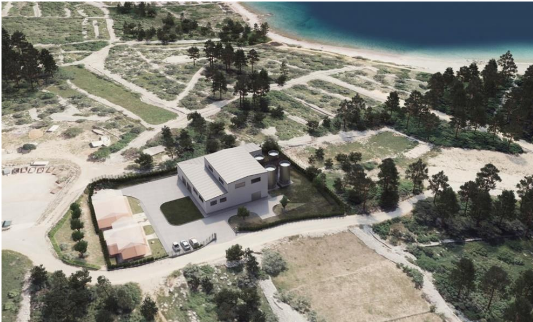
Figure 1: BAF Station with 10.000 PE in coastal area
