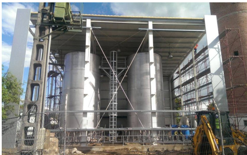
Figure 1: Biofiltration plant Targu Carbunesti with 2 biofilter during construction
