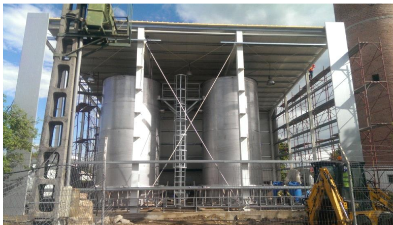
Figure 1: Biofiltration plant Targu Carbunesti with 2 biofilter during construction
